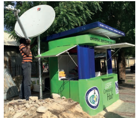
The 'Community Hub' is a dedicated comms block used for Gilat's Village Island system in each Nigerian village.
