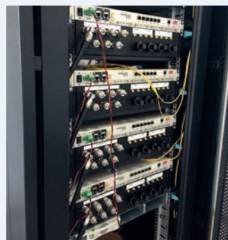
Dali's t-series equipment, including the RF Router , tHost headend, radio remotes and network management system, was used for the trial.
