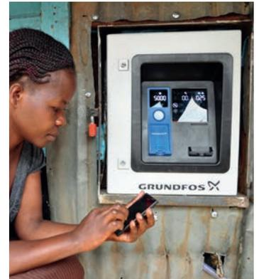
Grundfos' automated and connected water kiosks – known as water ATMs – dispense safe, clean water (left) and accept payment via *M-Pesa* (above).
