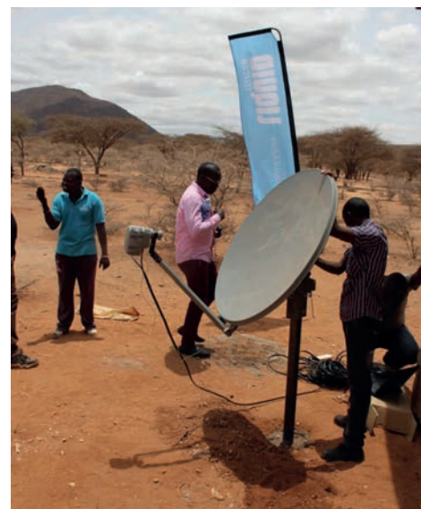
Liquid Telecom engineers install a VSAT dish on a one-metre high pole in the Kenyan village of Kiltamany.
