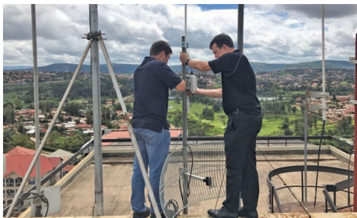
Engineers setting up Kigali's smart city LoRaWAN network.
