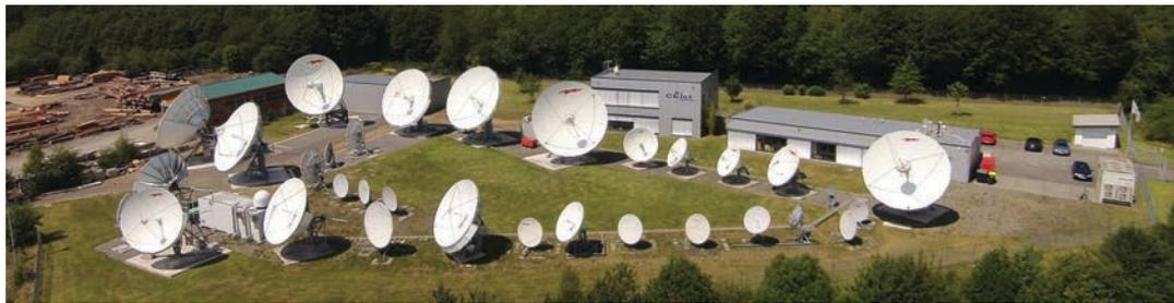
CETel's German teleport near Cologne and Bonn. The company says its antennas for standard C-band, extended C-band and Ku-band directly support geo-stationary and inclined satellites between 68°W and 75°E.
